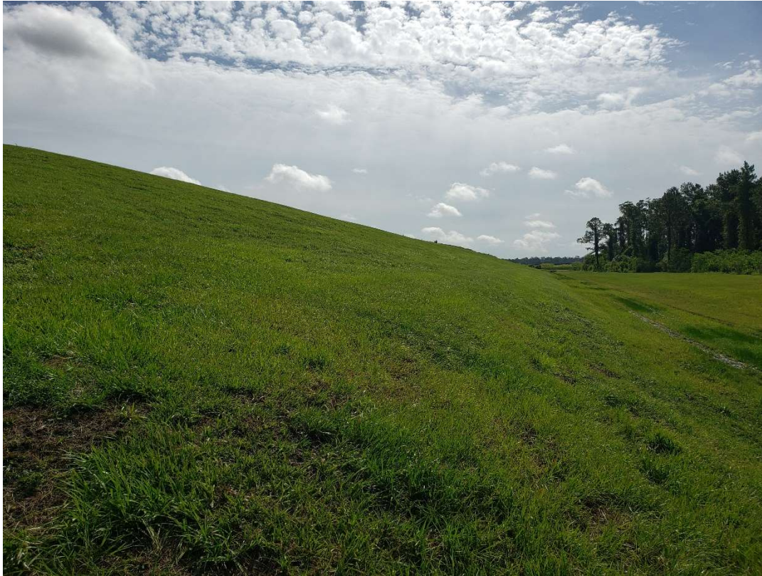
Figure A1. South Side of Landfill (No Ruts); 5/24/2022
