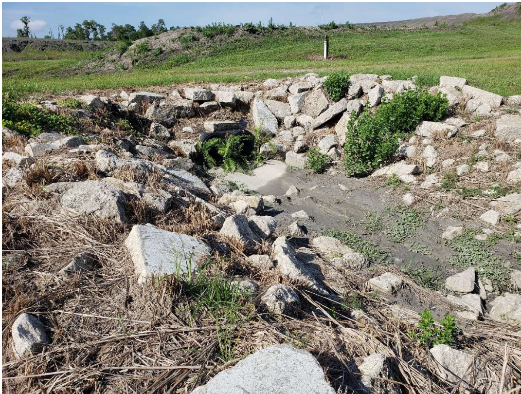
Figure A2. Cell 3 Culverts; 5/24/2022
